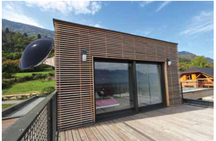
The water is heated directly and no pump is required
