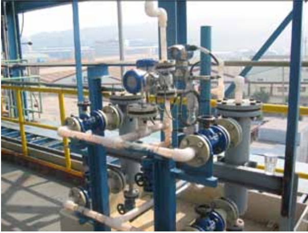
Figure 3 – OPTIFLUX 4300 with Virtual Reference shows the system in operation at Andritz
